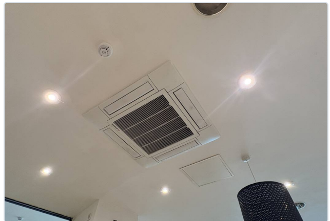
P12 — Seating-area ceiling
