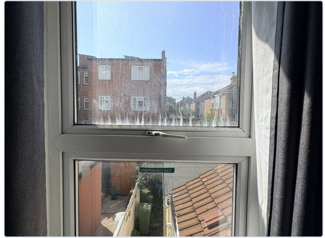
P18 — First-floor rear window
